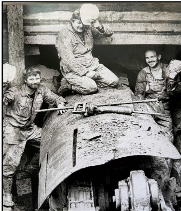
The hole through on the Titirangi Tunnels in 1989. Joe, left, was Site Manager. Jock Smith, Project Superintendent is on top with Grant Myocevich, the shift boss, right. A specialised small tunnelling machine was used for the 1.2m x 2.2m high tunnel.
