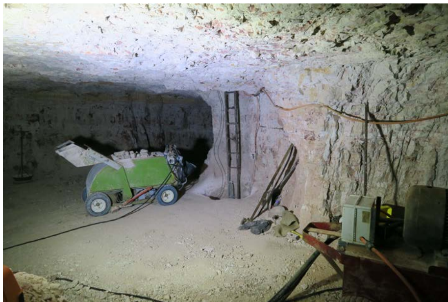
Figure 6: Hoist control unit (underground).
