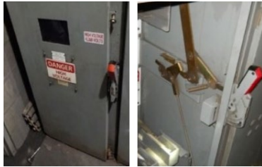
Linkage adjusted with circuit energized.
