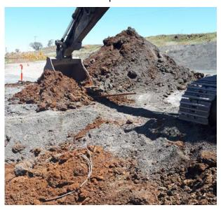
If the depth of cover is questionable, the depth should be confirmed before excavation begins. Any cables in the area should be isolated before starting to dig. Mines should keep surface infrastructure plans up to
