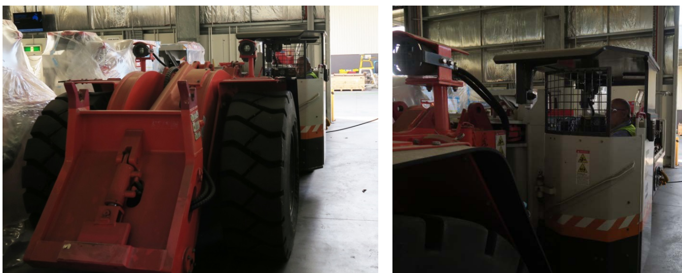
Figure 18: Guarding on a 7 Tonne LHD.
