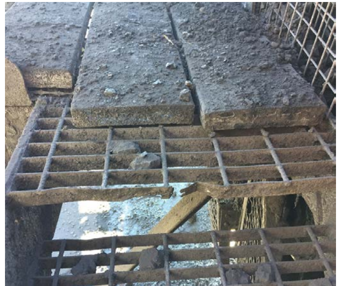
Figures 41 and 42: Significant corrosion of stair treads compromises structural integrity and creates trip hazard.
