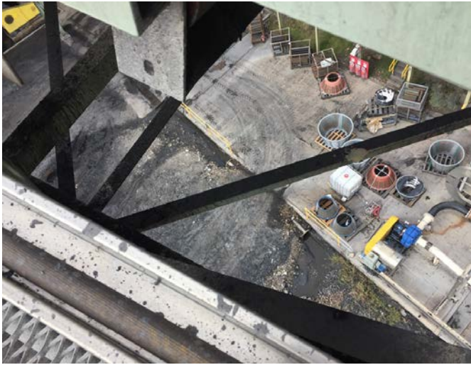
Figure 15: No protection to access road/storage area below. Figure 16: No protection if test weights dropped.
