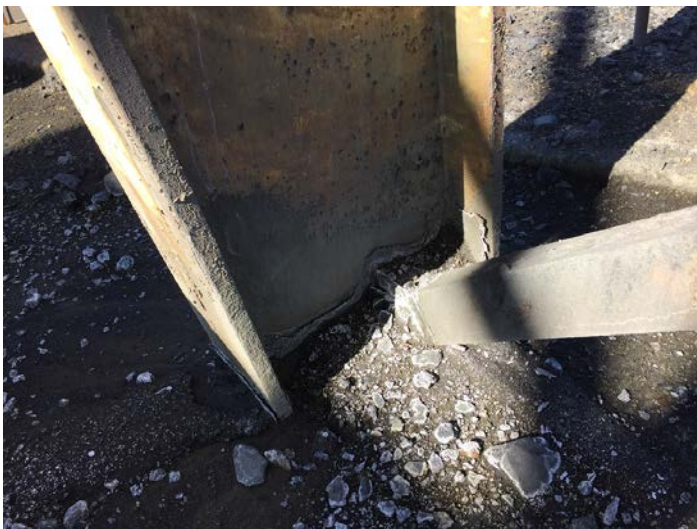
Figure 21: Corrosion of wall purlins.
