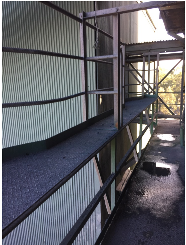
Figure 26: Platform added mounted to handrail.
