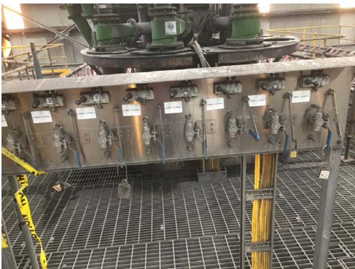
Figure 3: Pneumatic isolation board.
