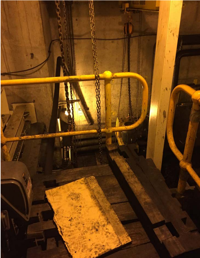
Figures 45 and 46: Rubbish, materials and scaffold boards become trip hazards, especially at the top of stairs
