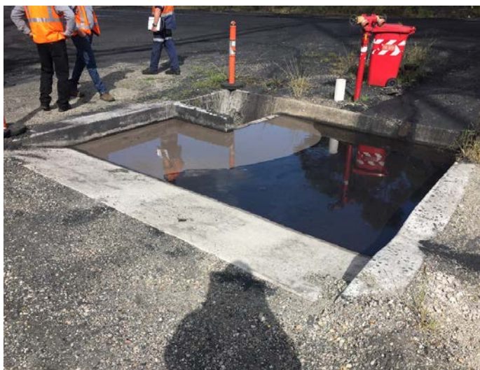
Figure 27: Sump with no protection or signs.
