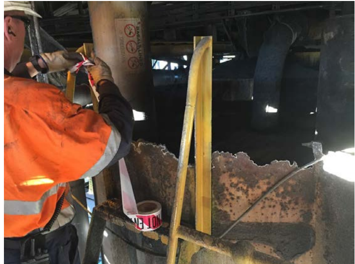
Figure 53: Door frame rusted through on both sides. Figure 54: Lip of dense medium sump corroded to a knife edge.
