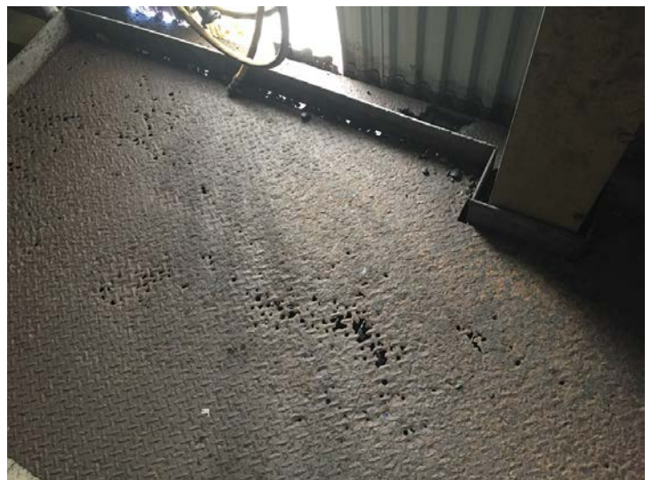
Figure 22: Full thickness corrosion of platform floor plate.
