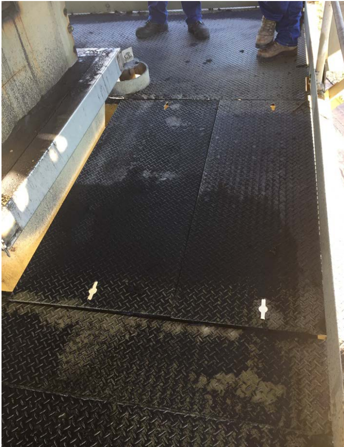
Figures 41 and 42: Significant corrosion of stair treads compromises structural integrity and creates trip hazard.
