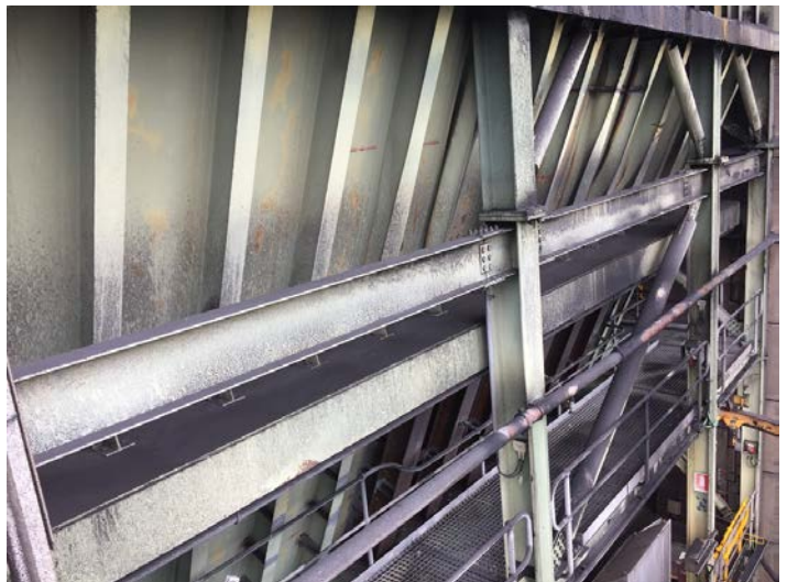
Figure 22: Full thickness corrosion of platform floor plate.
