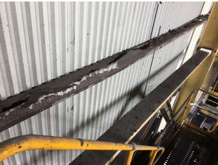
Figure 21: Corrosion of wall purlins.
