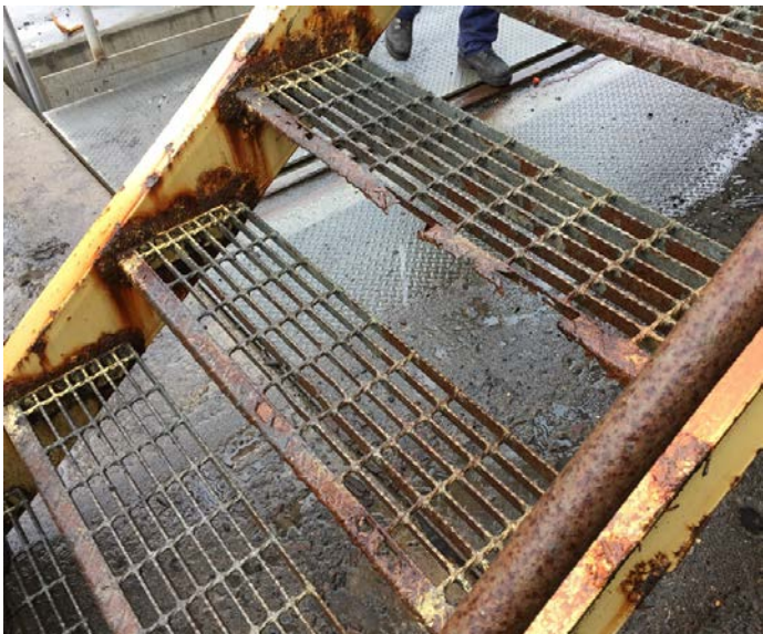
Figures 41 and 42: Significant corrosion of stair treads compromises structural integrity and creates trip hazard.
