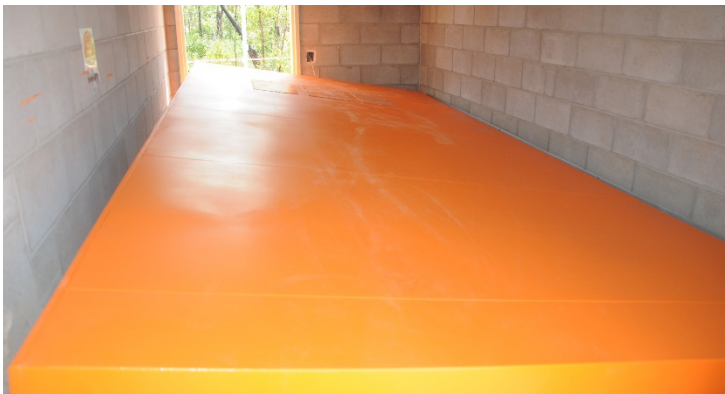
Image 2: The toppled over switchboard filling the room shows the workers were always at risk of being pinned.
