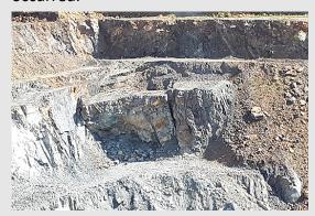
All mines with highwalls should complete geotechnical assessments to determine the design of the highwall. All geological and geotechnical issues need to be considered and highwalls designed accordingly.
