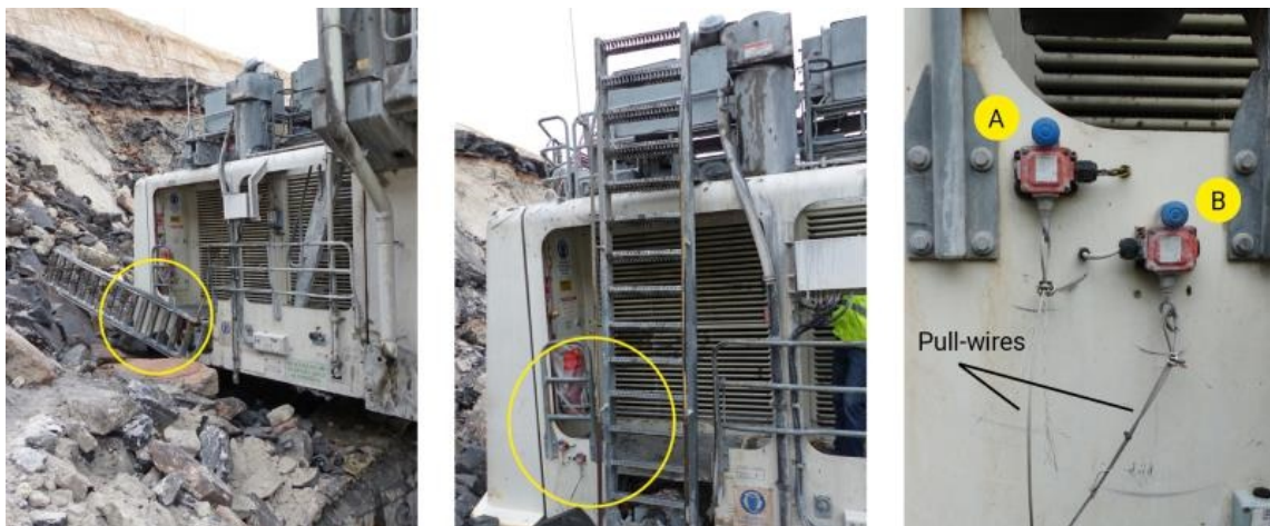
Circles indicate where the accident happened, showing the ladder in the final (left) and upright (middle) positions with the handrail, platform and emergency shutdown (A) and ladder (B) switches (close-up, right).
