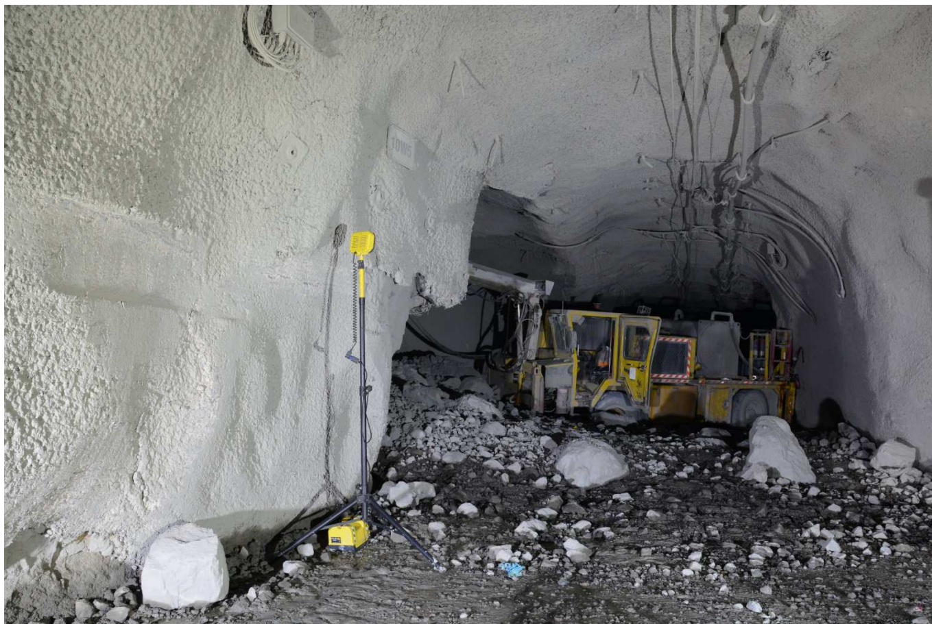
Figure 12 A photograph of the incident scene taken from the north side of draw point 6 in extraction drive 10, looking south (photograph by Department of Industry).
