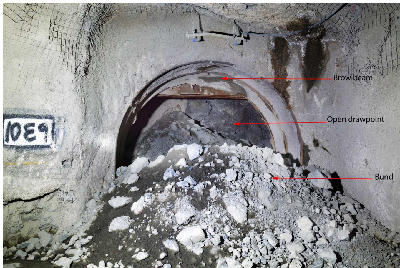
Figure 7 Photograph of 10E9 open, hung up draw point and bund.
