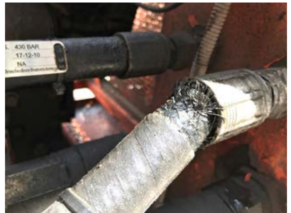
Figure 7: The failed hydraulic hose on the recovery power pack
