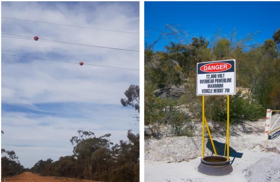
Examples of clearance indicators and signage for high voltage overhead powerlines
