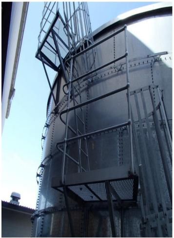
Photograph 1. Inclined caged ladder with additional rails installed to extend the height of the existing top guardrail.
