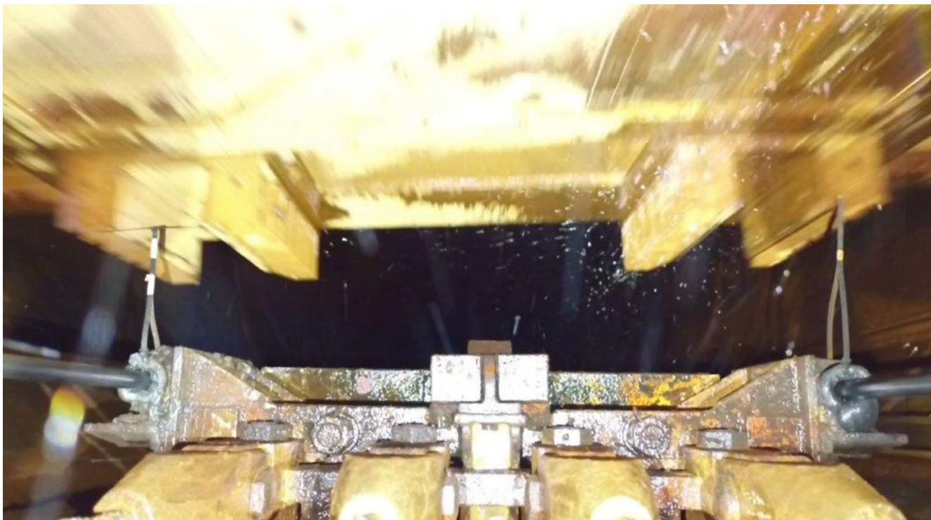
Figure 9: Counterweight to cage clearance.
