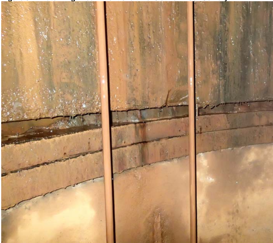
Figure 5. A water ring fixed in vent shaft No. 3 at Tahmoor Colliery.
