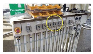
When he noticed no material on the belt he investigated to find that the locked-out conveyors had not started, and a considerable amount of material had built up at the transfer point between the feed belt and the isolated conveyors.
