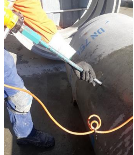
Re-enactment of worker core-drilling the concrete pipe
