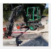
During a network burying operation, the excavator driver was about to move backwards with the machine. When he turned around to look at the area before backing up, his elbow hit the crane's joystick. The victim, who was in the machine's area of movement, was hit by the bucket on his right shoulder.
