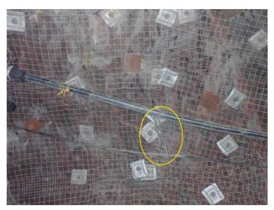
View of the failed chain installed to secure the air line to the backs.
