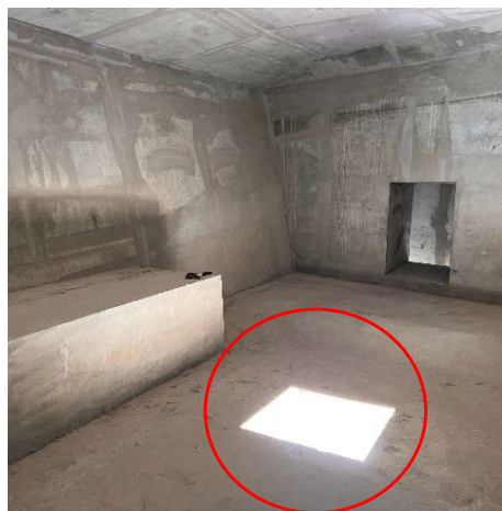
Opening in bottom slab within void
