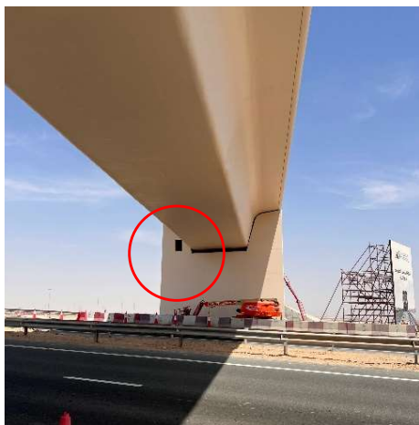
Access to hatch using MEWP
