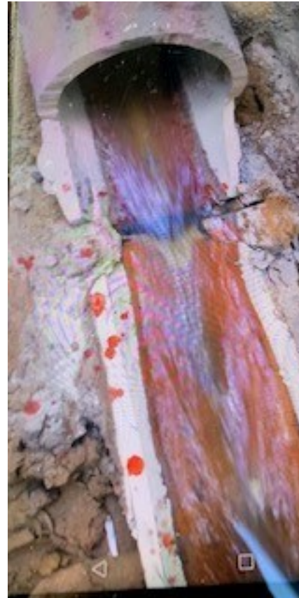
Section of pipe being cut with grinder
