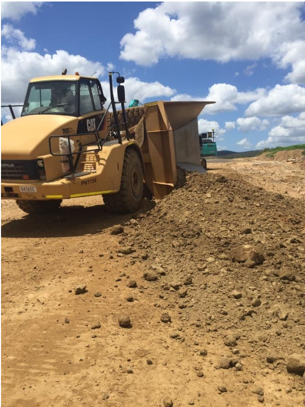
Photo 1 - ADT bin over
