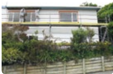
Figure 4: Scaffolding on a residential building.
