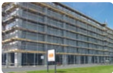
Figure 5: Scaffolding on a multi-storey building.
