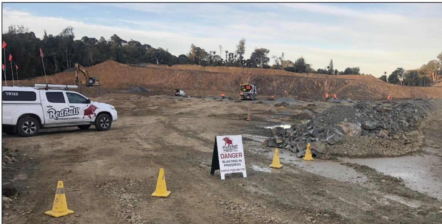
A risk assessment should be completed for each blast, identifying the hazards and controls at each stage, including the extent of the blast exclusion zone during the firing sequence. Any risk assessment and subsequent hazard controls should be agreed to and approved by all the relevant parties involved in the blasting process before blasting.
