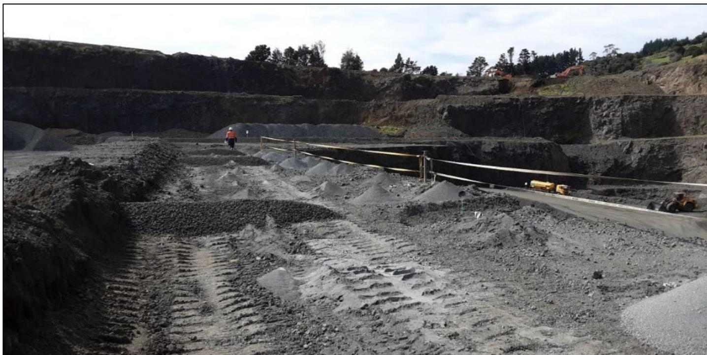
Bench preparation is critical in establishing a safe working environment for all activities associated with surface blasting. Standards for bench preparation must meet the requirements of subsequent on-bench activity, in terms of the preparation and demarcation of those areas.
