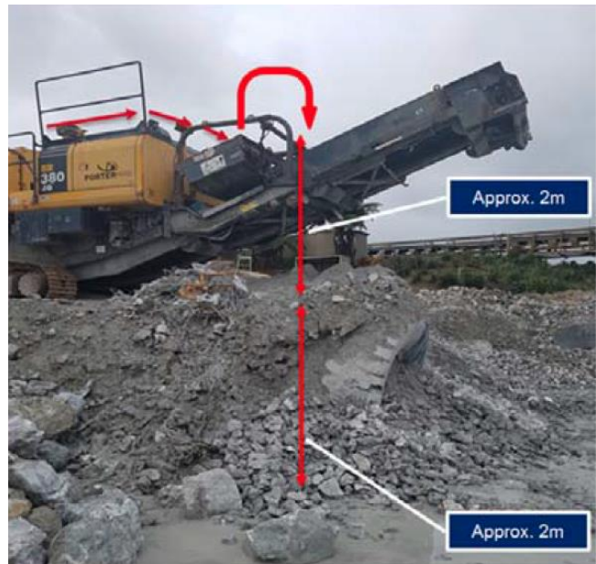
Indication of fall height from crusher
