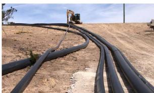
When poly pipe is being moved, the stored energy and potential for sudden release (spring back) must be taken into account in task procedures. Clear and defined 'no-go' zones must be developed to protect workers from sudden releases of energy.
