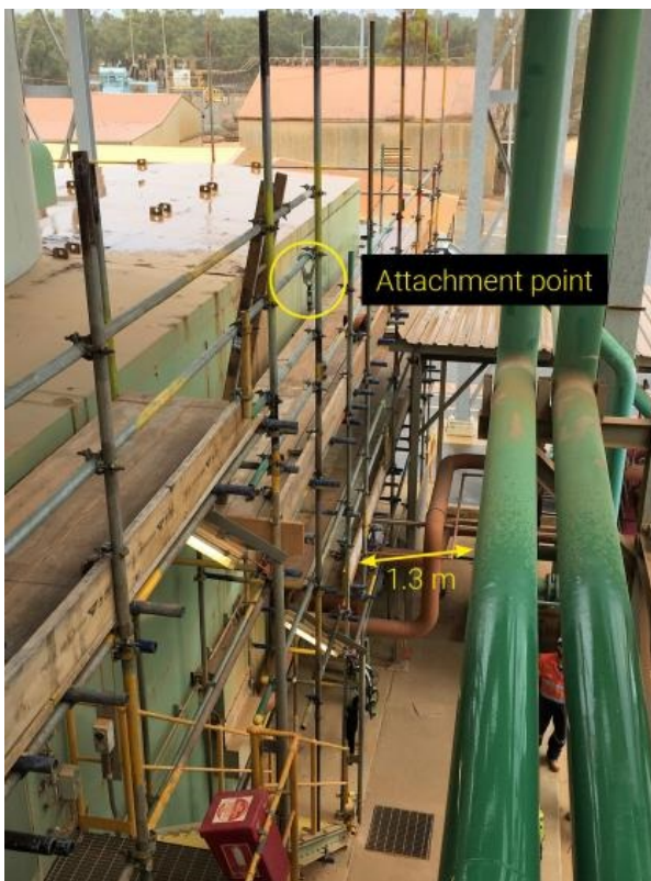
Left: Void between scaffold and pipe support structure. Right: Fall location and height.
