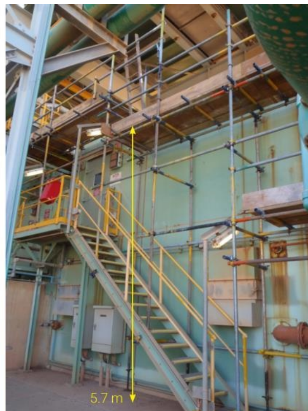
Left: Void between scaffold and pipe support structure. Right: Fall location and height.
