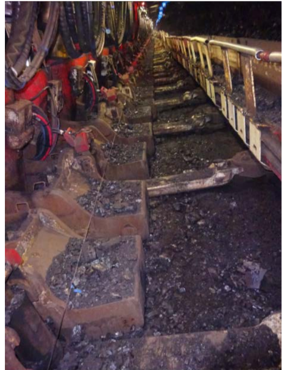
Figure 2: Ejected coal in the walkway as a result of the coal burst. ii
