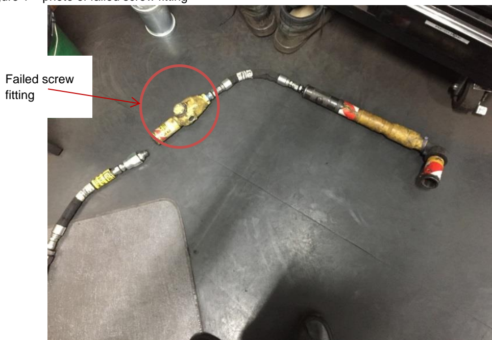
Figure 1 – photo of failed screw fitting
