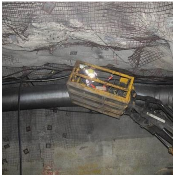
IT work basket in position beneath the backs
